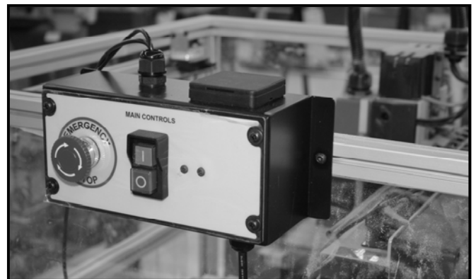
Figure-3 Installing the switch box
