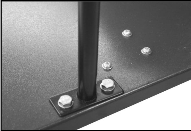
Figure-7 Installing the collector ring support
